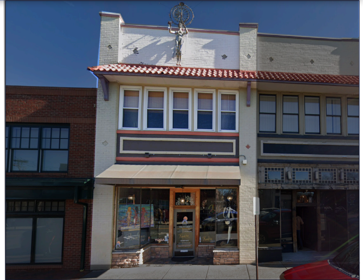
First Floor Retail
